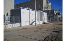
and operated continuously under 100% rated electrical power output for up to 240 hours. The enclosure integrates IBC-rated seismic restraints to 1.5, can withstand maximum wind loads of 150 mph, 50-psi roof loads, 250-psi floor loads, and endure temperature extremes from -30°F to 120°F.
