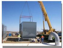
three generator sets (gensets)—Diesel engines mated to generators and power controls, and placed within weatherproof steel enclosures equipped with integral fuel tanks for storage of No. 2 Diesel fuel oil, to power the generators.
